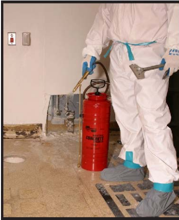
Using a tank sprayer to wet seams
