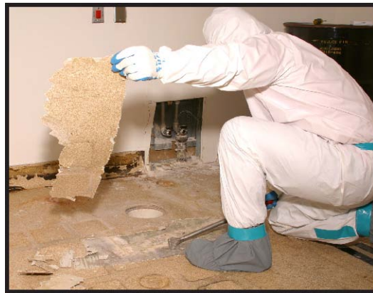
Lifting up and removing a section of flooring
