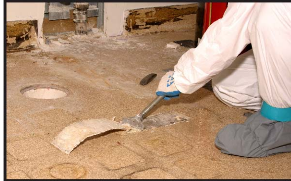
Using a hammer and chisel
