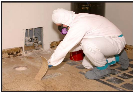
Prying up a section of flooring
