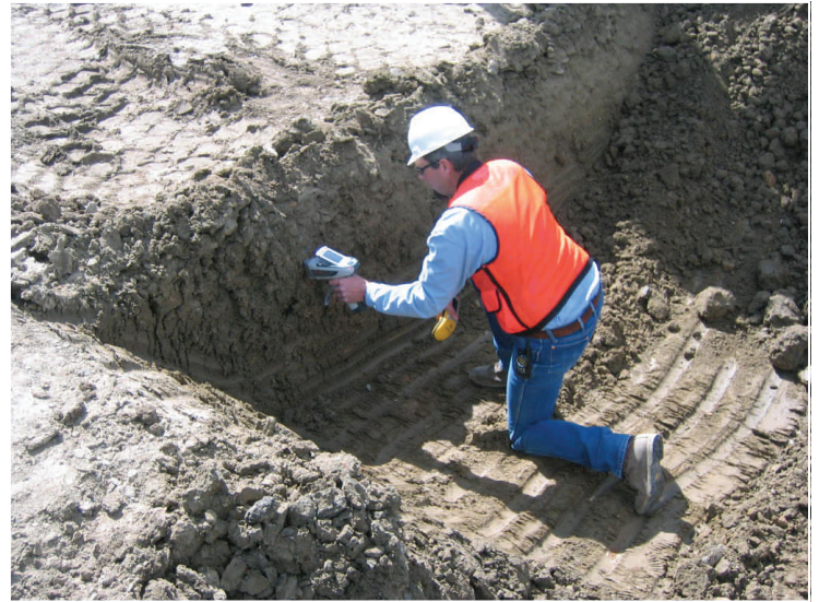
Field screening excavation side walls
