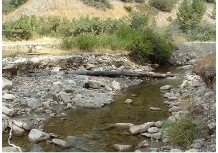
Exposed pipeline in Beaver Creek north of Nelson, MT
