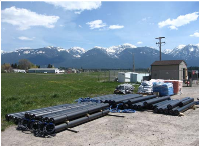
Phase III ERH Installation
