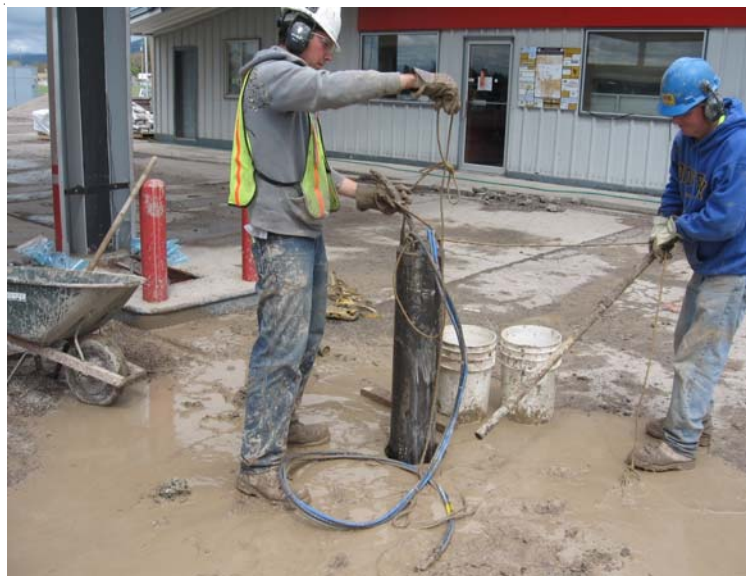
Electrical Resistance Heating Installation continued on page 5
