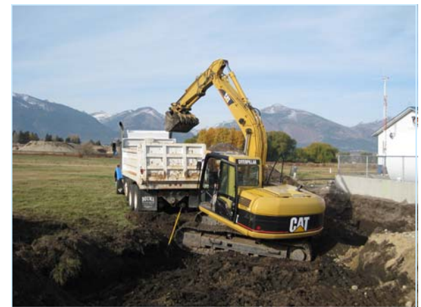
Ravalli County Airport jet fuel spill excavation, October 2008.
