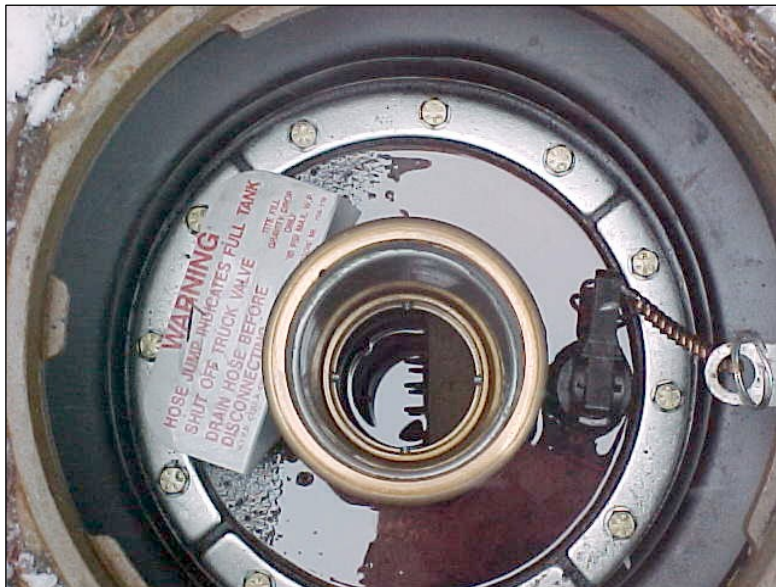
Looking down a fill pipe at a flapper valve
