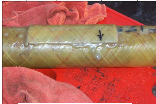
Repaired FRP Piping
