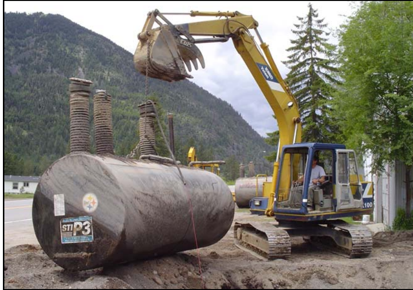
Permanent Closure – Tank Removal
