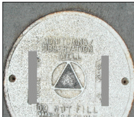
Sample Monitoring Well Cover
