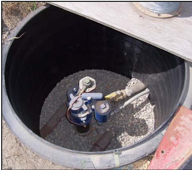
Sample Sump of a Pressurized System
