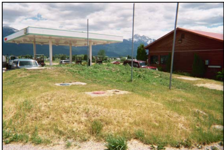
Tank Nest and Vent Stacks
